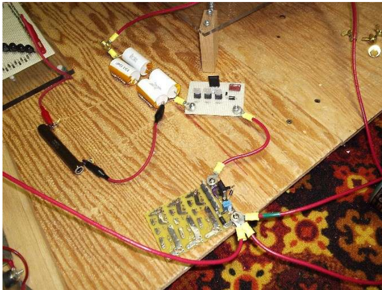
Figure 13. First coil setup with two prototype 900V sections.
